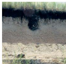
Fig. 1.4: Pit in the river embankment at the Likwala-aux-Herbes, Km. 186 (LKW 87/186).
