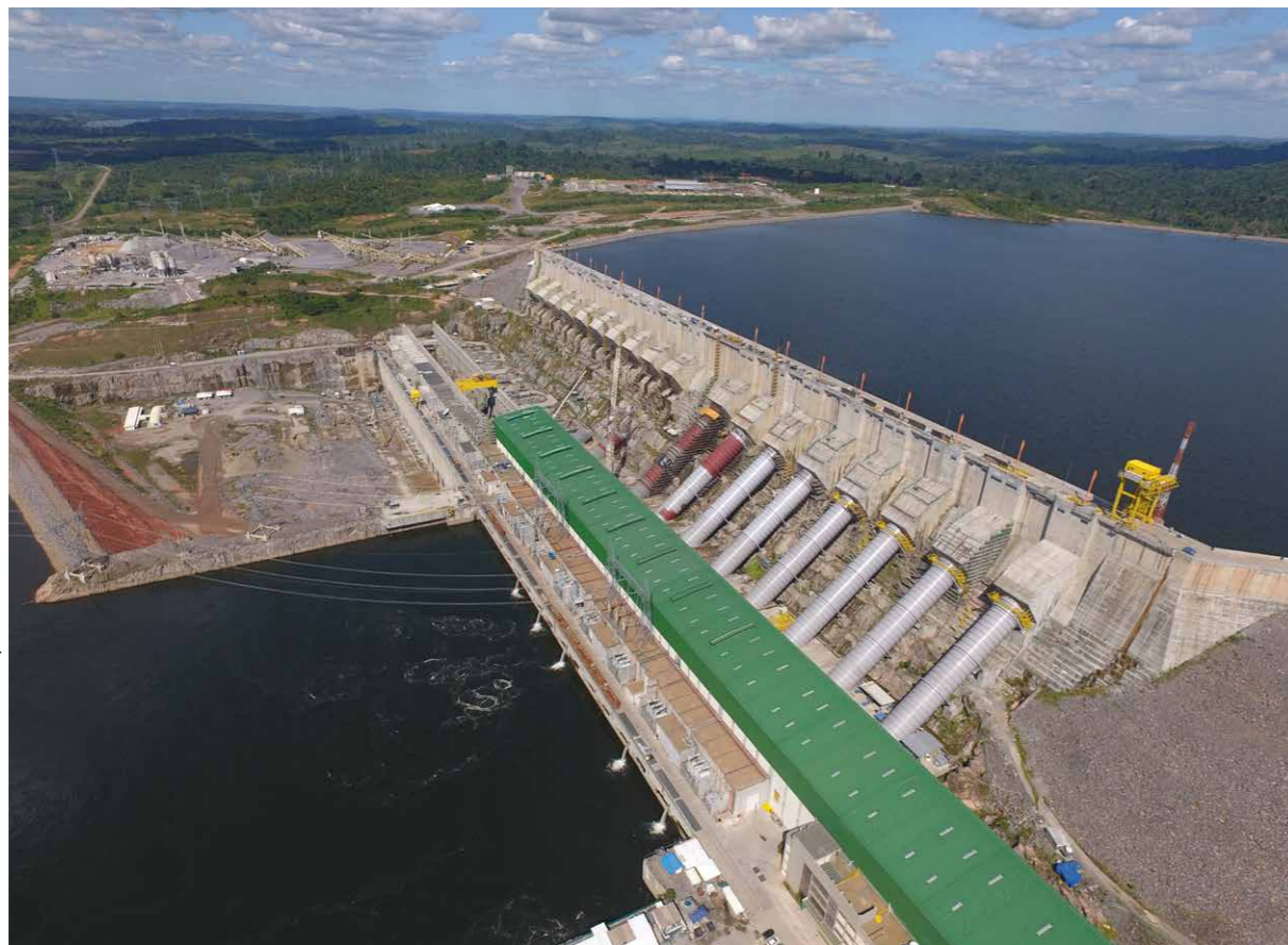
FIG 1 Belo Monte dam in the Xingu Basin of the Amazon. This was the third largest dam in the world at the time it was completed in 2016. It has an installed capacity of 11 GW but many months a year it produces only 4 GW, and in July to November of 2022 it was unable to produce any energy at all due to low water levels. Most of its energy serves distant cities and industries in Southeast Brazil.
